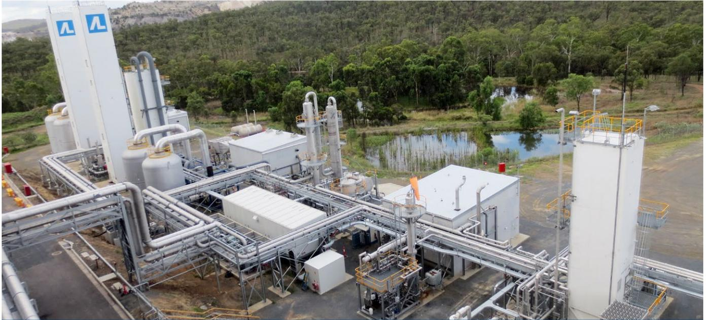
The completed air separation unit and carbon dioxide processing unit on the Carbon Dioxide Capture Plant.
