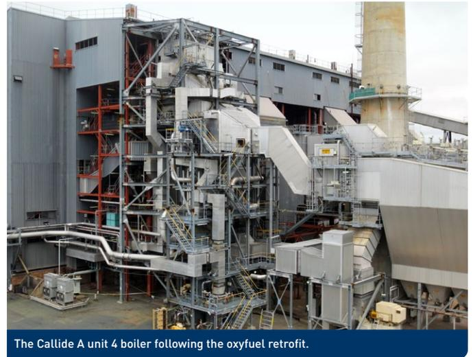
The Callide A unit 4 boiler following the oxyfuel retrofit.
