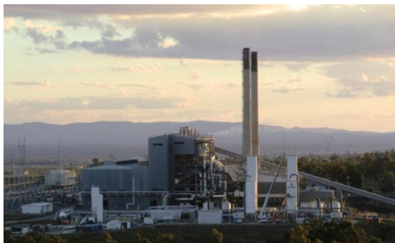
Fig. 5. Side view of Callide A power station
