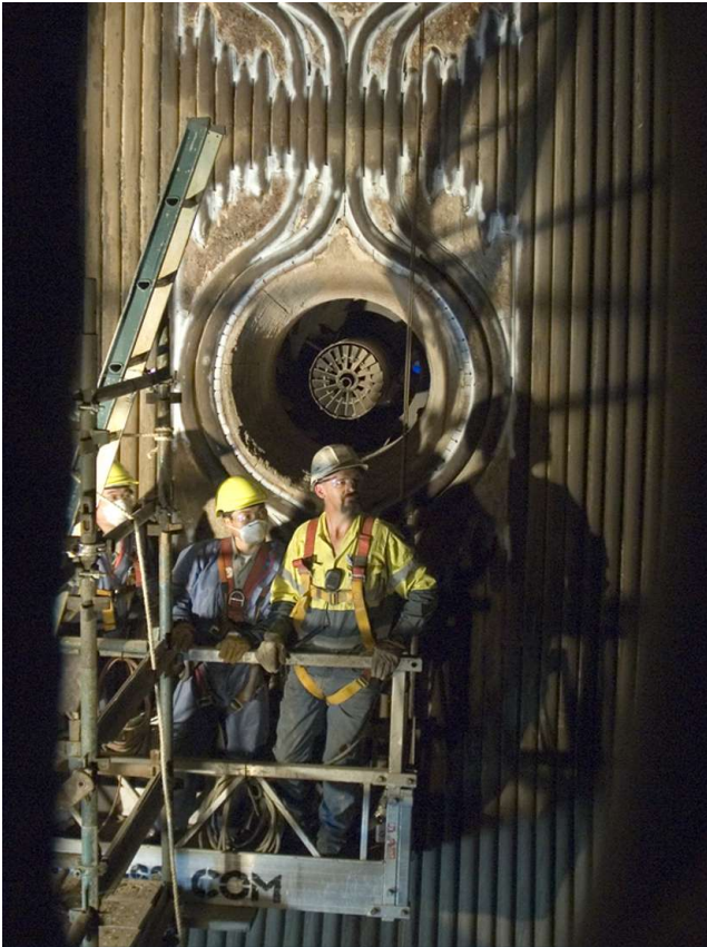
Inside the Callide A furnace during the condition assessment in October 2006.
